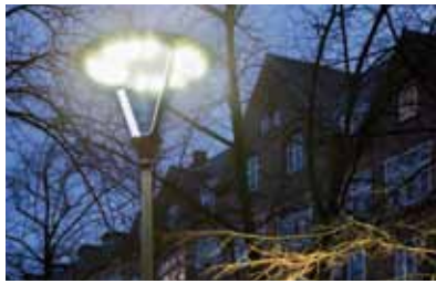
UrbanScene LED lights efficiently light square.
